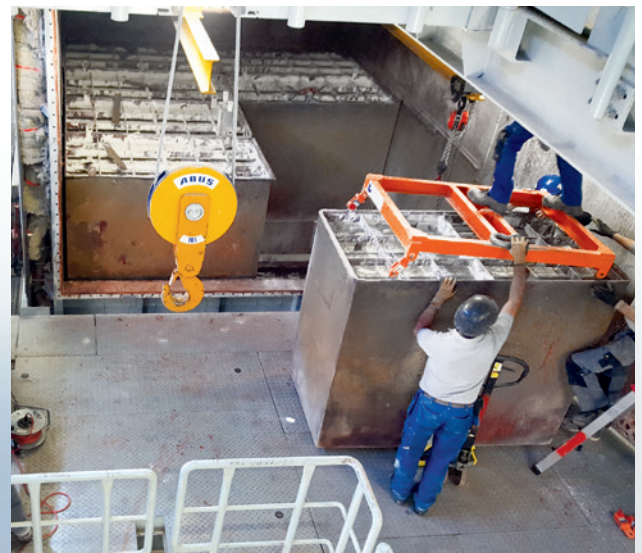
Catalyst installation
